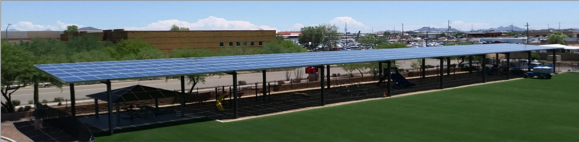
Elevated solar shade structure – Playground
